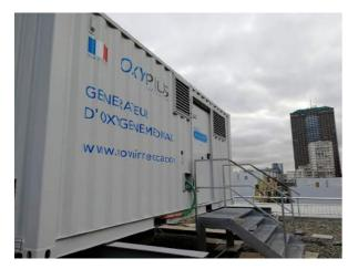
Caption: Containerized PSA oxygen plant installed on the roof of La Roseraie Hospital near Paris, France
