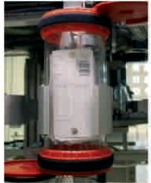
TranspoNet, the Pneumatic Tube System delivers therapy rings automatically to the wards
