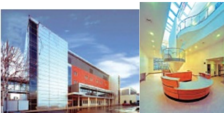
Computer simulation of Belfast City Hospital's new oncology building.
